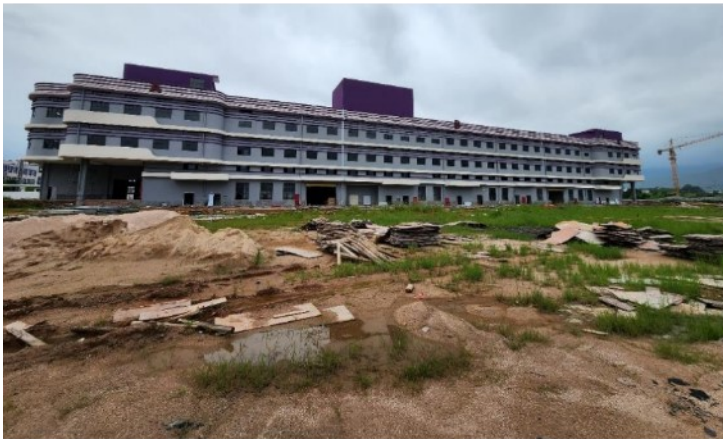
Infrastructure for high-tech manufacturing facility, research laboratories, and office.
