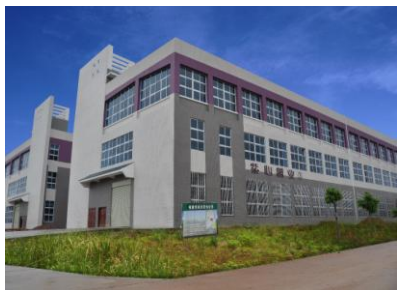
Completed factory of Fujian Zilaohu in Liancheng Industrial Park, Food Processing Area will be operational by end of 2016.
